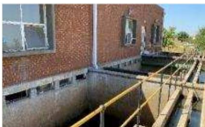
Standerton WTW rapid gravity filters
