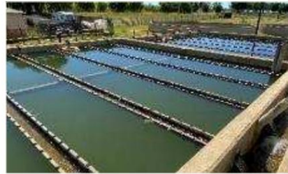
Standerton WTW settling tanks
