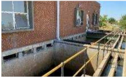
Standerton WTW rapid gravity filters
