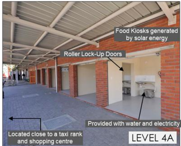
Cape Town - Nomzamo Business Area
